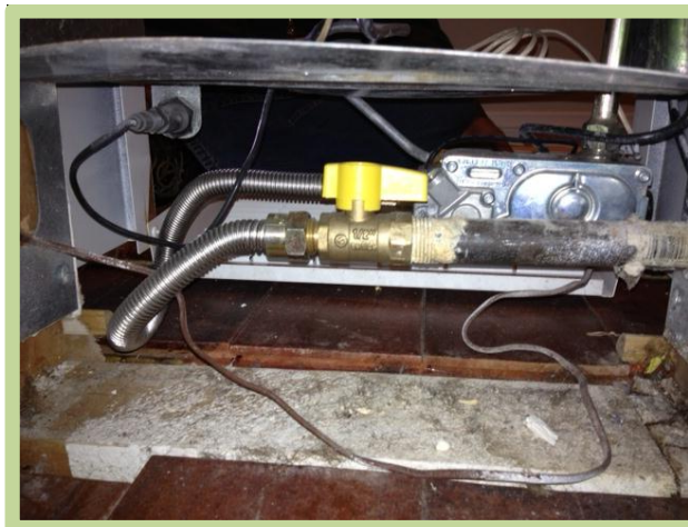
Furnace Line Valve and Flex Connector
