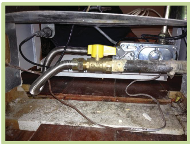
Furnace Line Valve and Flex Connector
